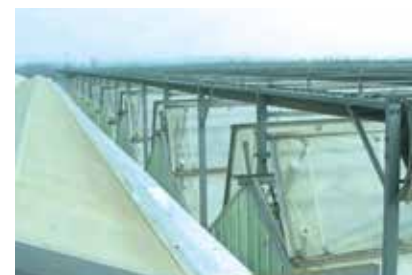
二分之一开窗 1/2 fully opened roof system
