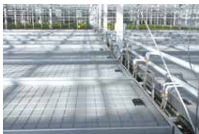
潮汐式灌溉苗床 Ebb-and-flow irrigation system
