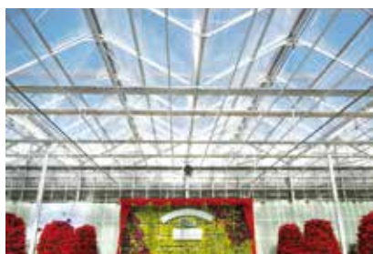
ETFE 膜双屋脊大跨度新型温室结构 New-type greenhouse structure with ETFE film, large-spanned double ridge structure
